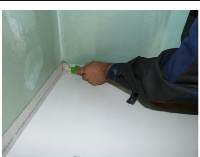
06: Waterproofing the shower tray with Aquaproof sealing collar.
