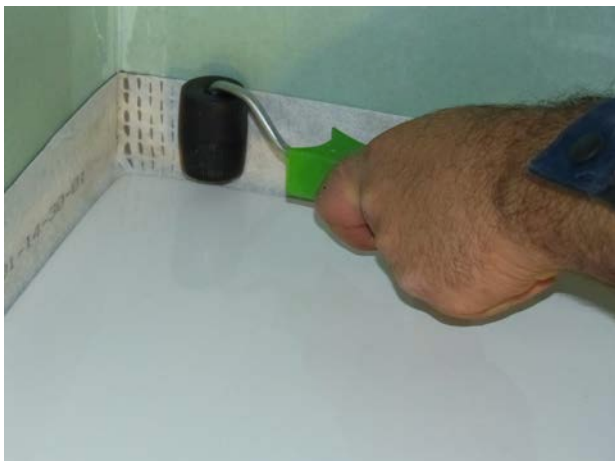
07: Corner areas can be waterproofed particularly well with Aquaproof bathtub/shower tray sealant strip.
