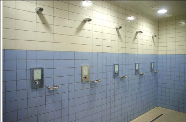
10: The Schell wall installation shower Linus at the Seebad pool in Schorndorf is equipped with a radar sensor system: It registers the presence of the guest and automatically stops the flow of water as soon as they leave the sensor area. The water keeps running for another 5 seconds to ensure that any soap residue is fully removed.
